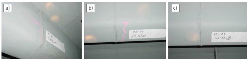
Figure 1. Fatigue cracks in butt welds of longitudinal ribs (cracks are marked with pink lines) [10]
