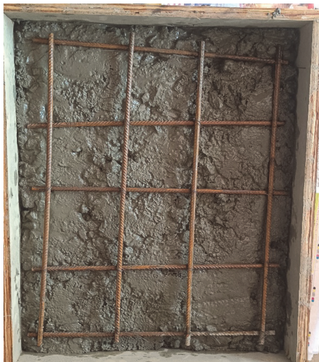
Figure 3. Casting conventional concrete slab
