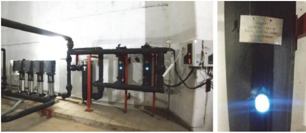
Figure 8. Building rainwater UV treatment system
