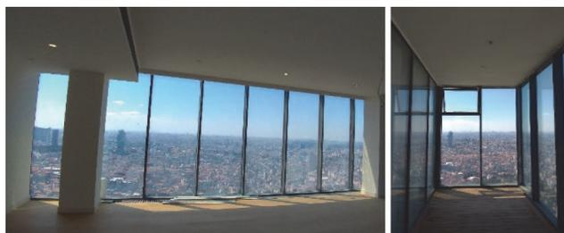
Figure 4. Photographs demonstrating insufficient number of operable windows on the façade
