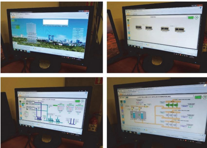
Figure 10. Building control centre automation system
